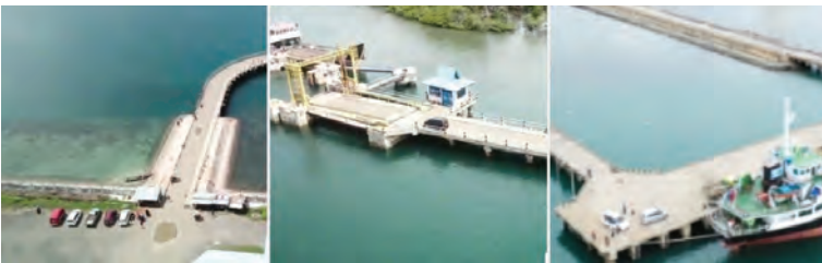
The Sorong SEZ area which ends at the SEZ port. (PHOTO/SRc)/dok).
