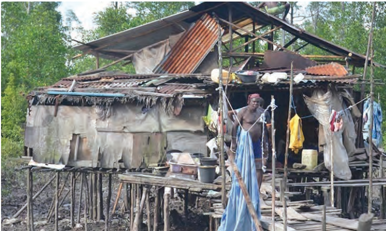
HOUSE - The condition of longginus Ainiu's house in Pomako. Photo: Kristin Rejang/ Seputarpapua.
